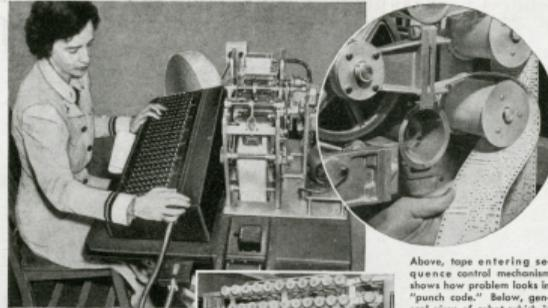
Solving problems which stumped mathematicians throughout history, is all in the day's work to the "world's greatest calculating machine" which gives accurate answers in 23 figures. Above, preparing a problem for the machine on manual tape punch which dictates operation of the "superbrain" with coded perforations. Center, system of holders on which tape moves
